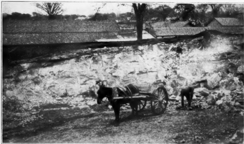
Dump Cart Hauling Stone to Crusher. Note Thin Top Soil
